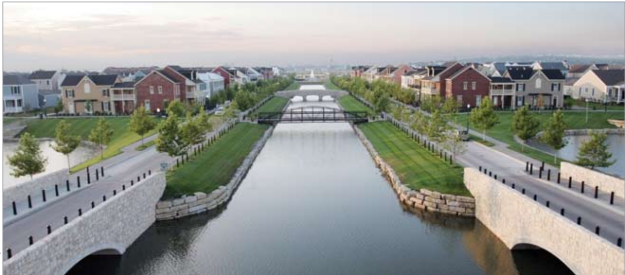
Courtesy of the New Town at St. Charles
